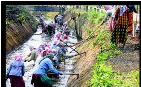
Mahatma Gandhi National Rural Employment Guarantee Scheme workers engaged in cleaning the left bank channel of the Karapuzha Irrigation project in Wayanad
